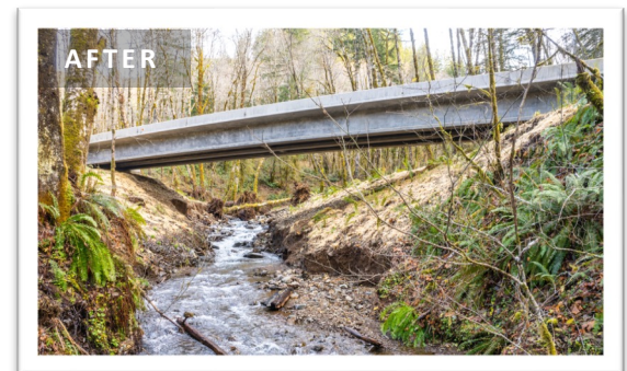
AFTER: The new 115 ft bridge allows conveyance of high flows, wood, and sediment.
