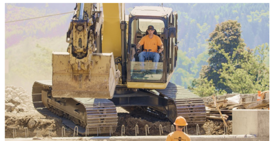
Placing boulders to protect the bridge footings.
