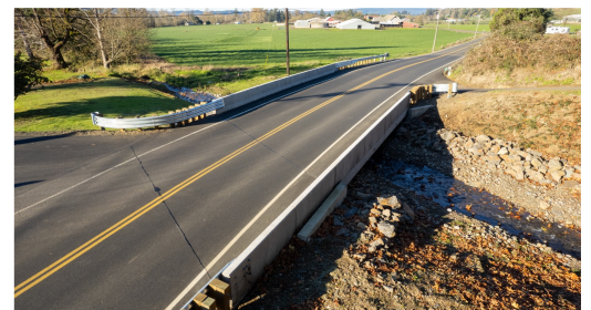
Placing boulders to protect the bridge footings.
