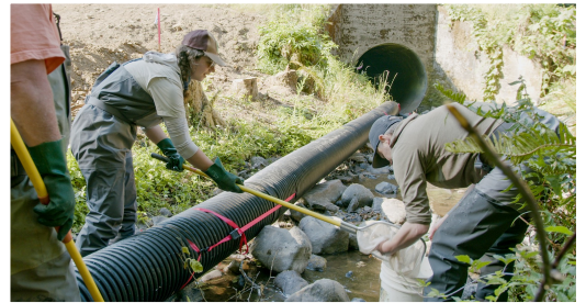
DURING: Aquatic species are moved to safety before construction begins
